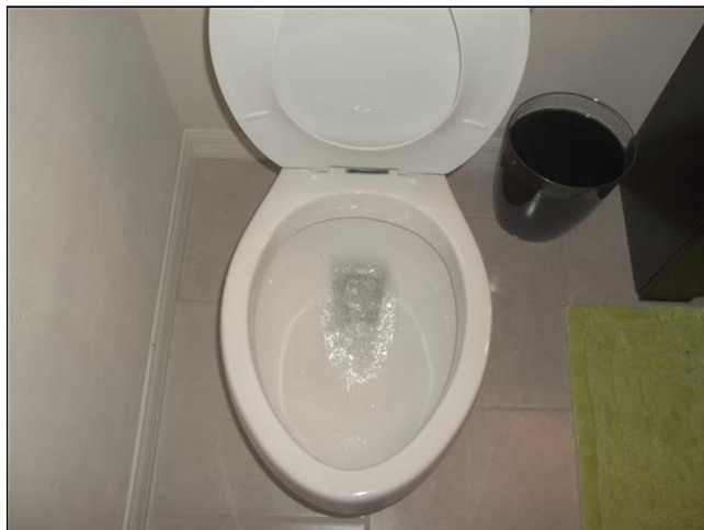
6.0 Item 2(Picture) Toilets
