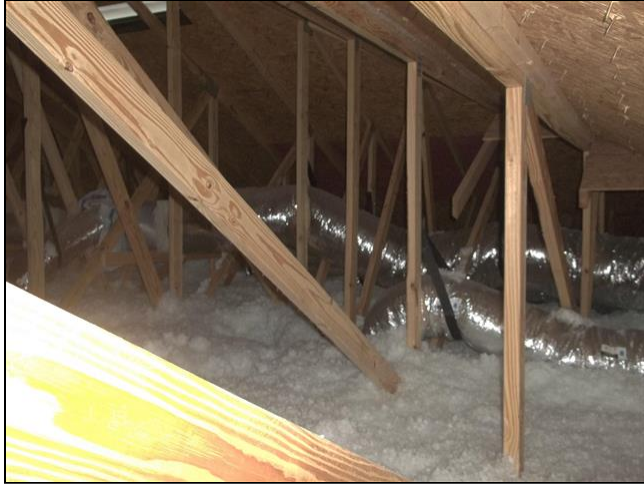
8.3 Item 1(Picture) Duct Work
