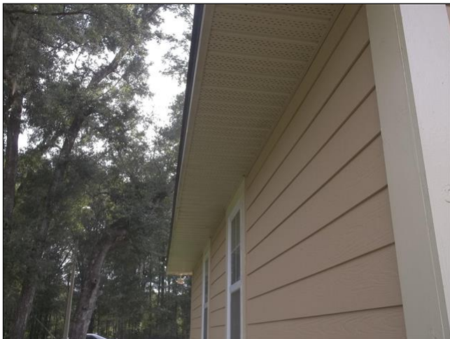
2.5 Item 3(Picture) Soffit
