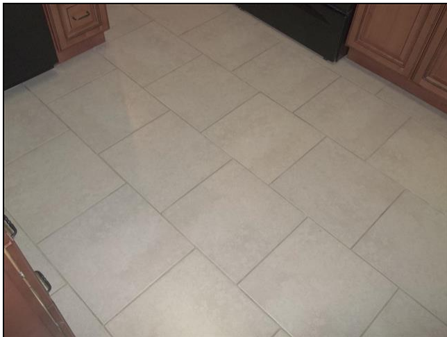
4.2 Item 1(Picture) Floors
