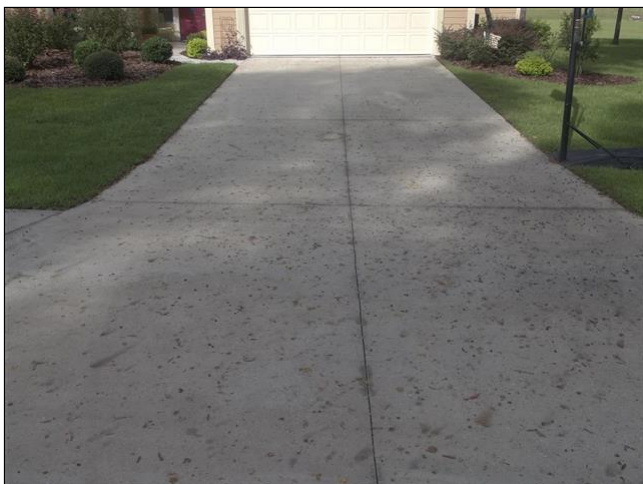
2.3 Item 5(Picture) Drive way
