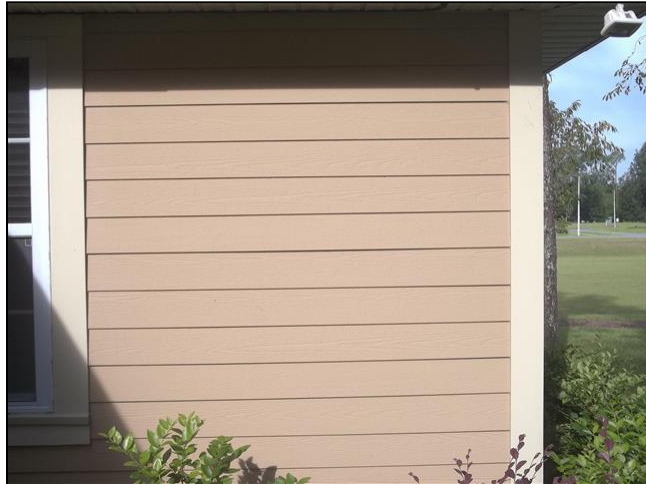
2.0 Item 1(Picture) Siding
