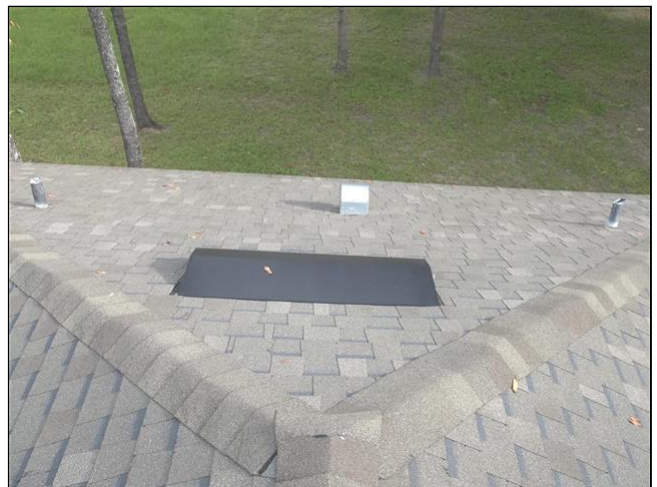
1.2 Item 6(Picture) Roof Penetrations
