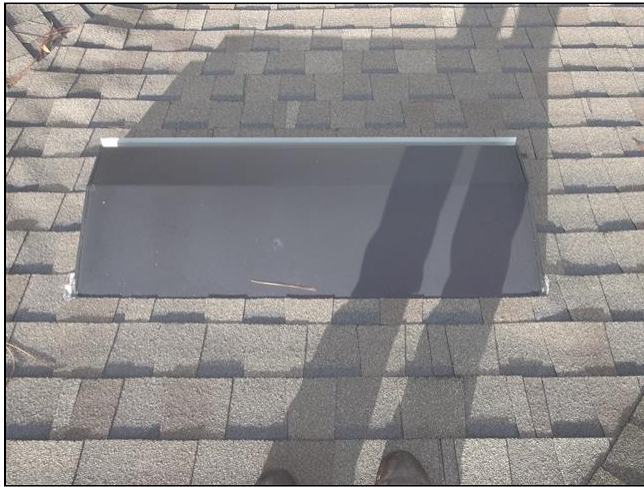
1.2 Item 1(Picture) Roof Penetrations
