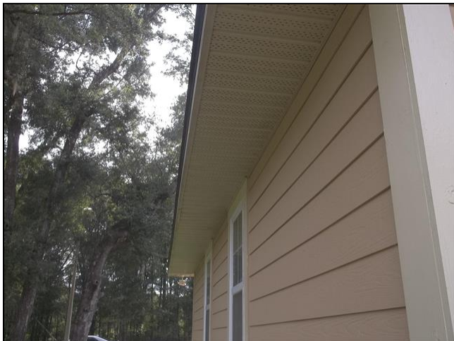
2.5 Item 3(Picture) Soffit
