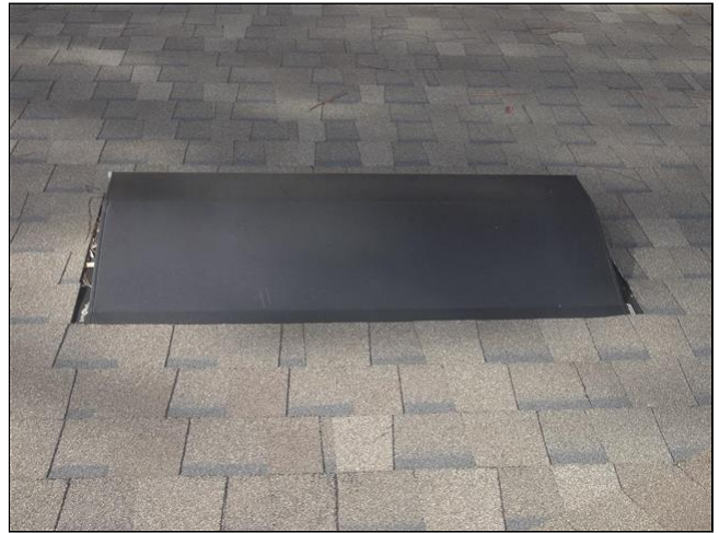
1.2 Item 2(Picture) Roof Penetrations
