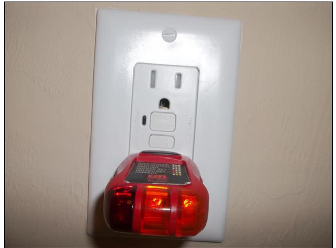
7.5 Item 2(Picture) GFCI's
