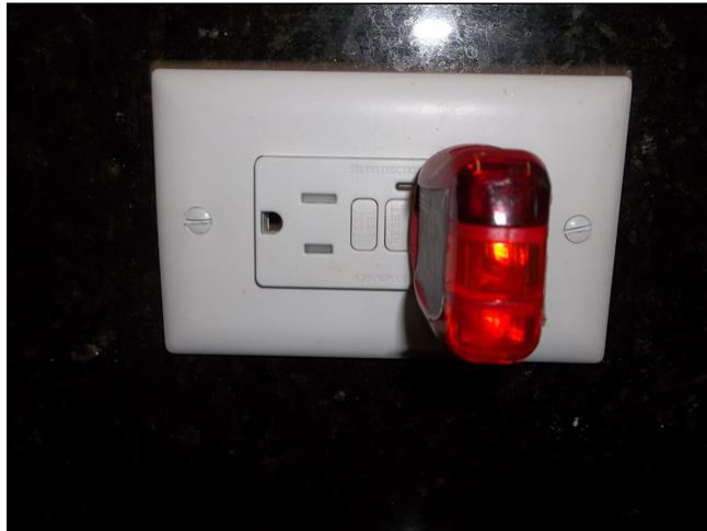
7.5 Item 1(Picture) GFCI's
