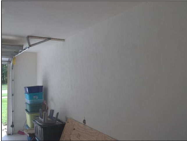
3.1 Item 1(Picture) Garage Walls
