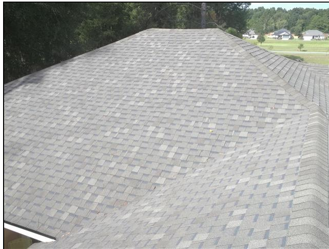
1.0 Item 1(Picture) Roof
