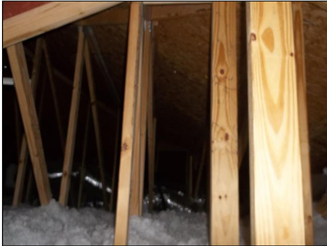
5.1 Item 1(Picture) Attic
