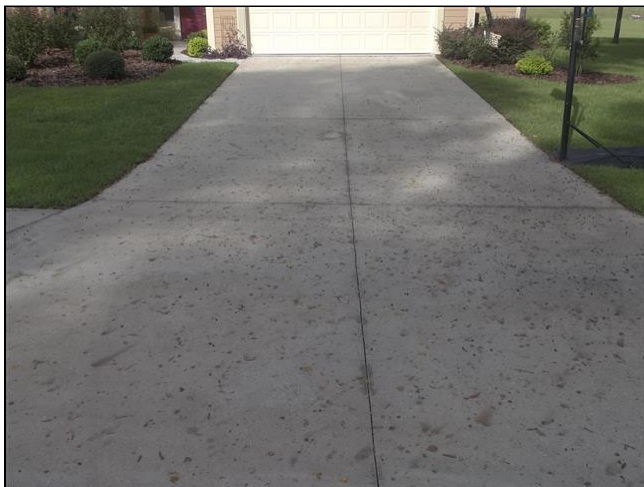
2.3 Item 5(Picture) Drive way
