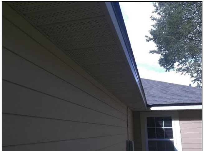
2.5 Item 2(Picture) Soffit
