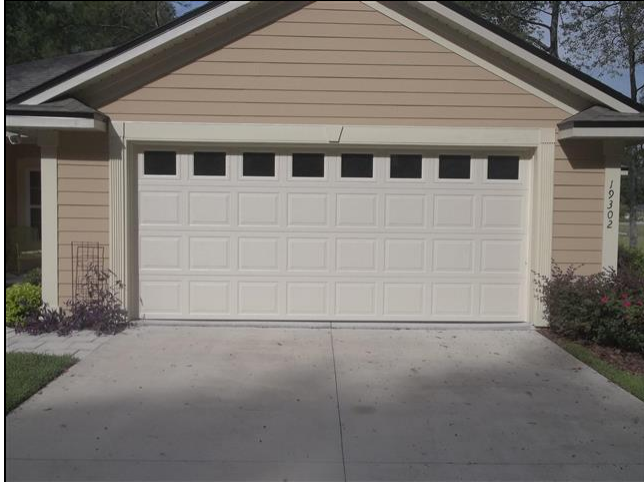
3.3 Item 1(Picture) Garage Door
