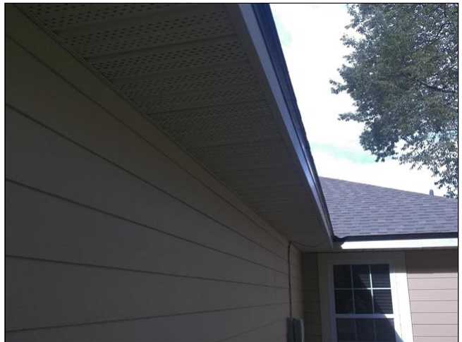
2.5 Item 2(Picture) Soffit
