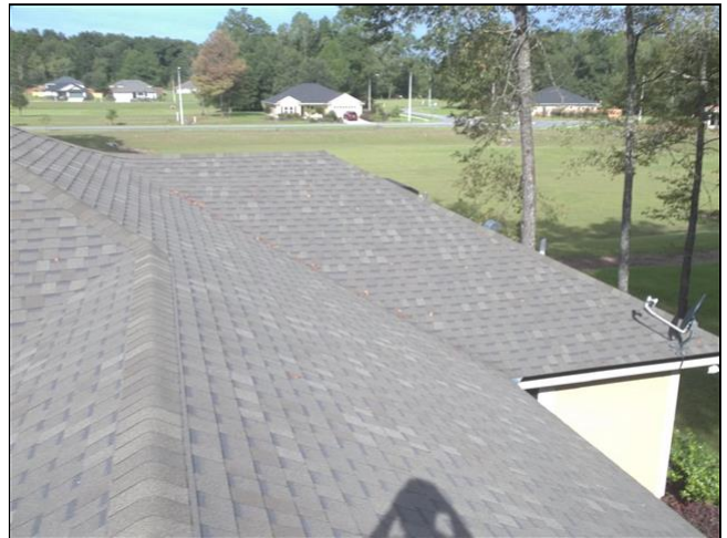
1.0 Item 2(Picture) Roof
