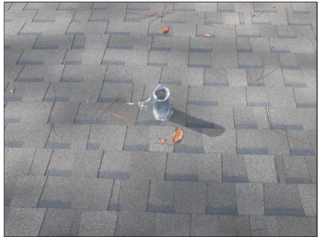
1.2 Item 4(Picture) Roof Penetrations
