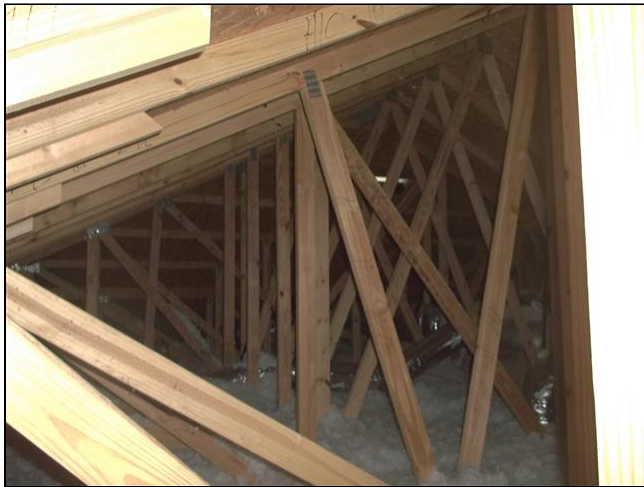
5.1 Item 3(Picture) Trusses
