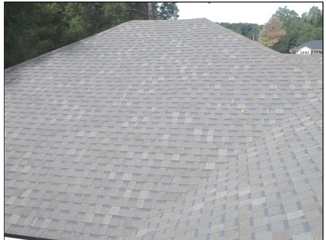
1.0 Item 4(Picture) Roof
