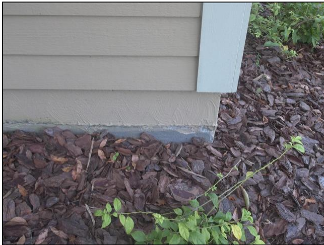
5.0 Item 1(Picture) Foundation
