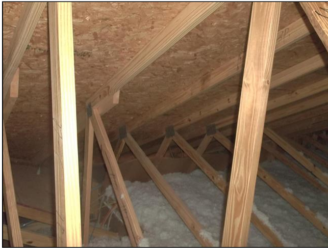
9.0 Item 1(Picture) Insulation in Attic
