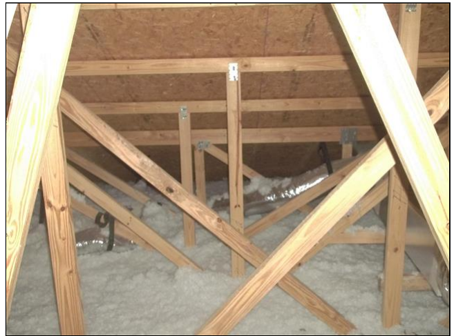
5.1 Item 4(Picture) Attic
