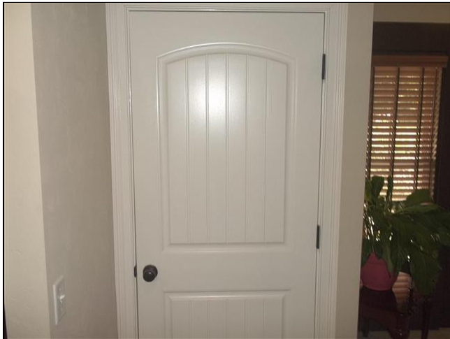
3.4 Item 1(Picture) Occupant Door
