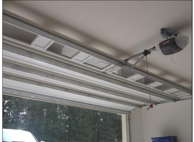
3.3 Item 2(Picture) Garage Door
