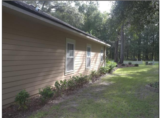
2.0 Item 2(Picture) Siding
