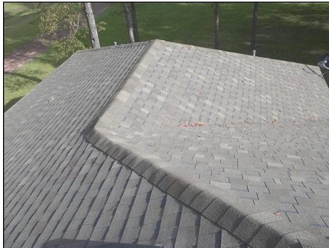
1.0 Item 3(Picture) Roof
