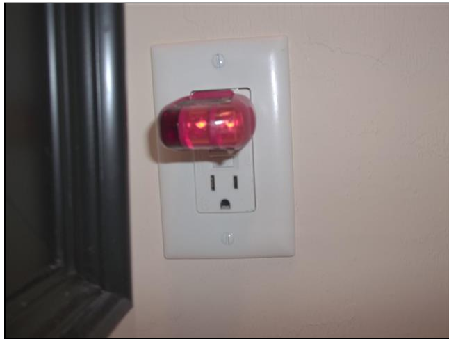
7.5 Item 3(Picture) GFCI's
