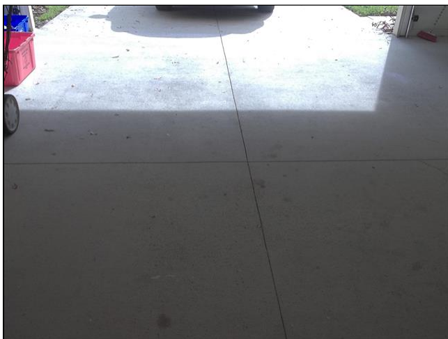
3.2 Item 1(Picture) Garage Floor
