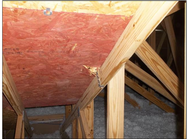
5.1 Item 2(Picture) Roof Decking
