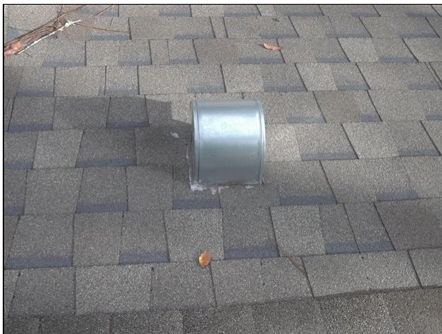
1.2 Item 5(Picture) Roof Penetrations
