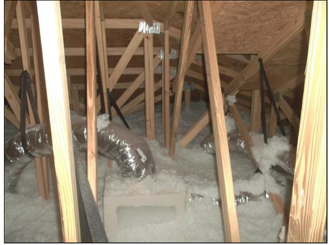
8.3 Item 2(Picture) Duct Work
