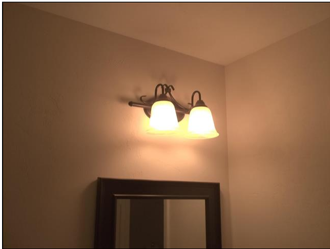
7.3 Item 3(Picture) Lighting
