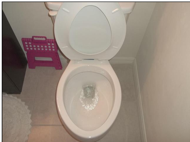
6.0 Item 1(Picture) Toilets
