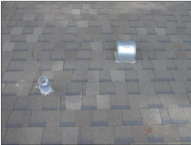
1.2 Item 3(Picture) Roof Penetrations
