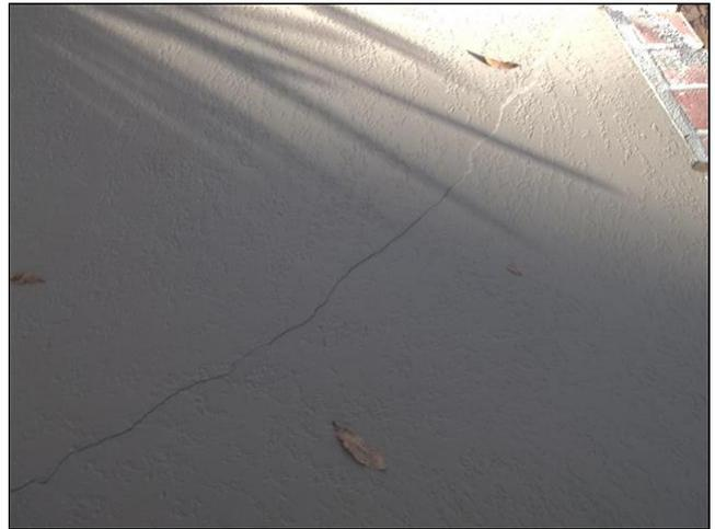
2.4 Item 4(Picture) Evidence Of Step Cracking
