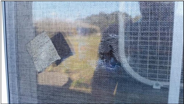
2.2 Item 1(Picture) Damaged Screen
