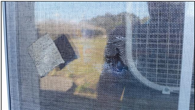
2.2 Item 1(Picture) Damaged Screen
