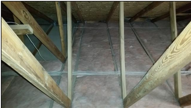
9.0 Item 1(Picture) Attic Insulation
