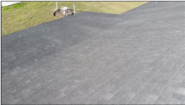
1.0 Item 3(Picture) Roofing
