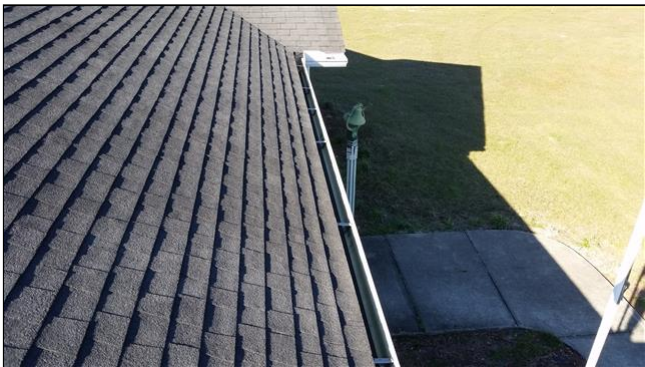
1.3 Item 2(Picture) Roof Drainage System
