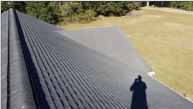
1.0 Item 2(Picture) Roofing
