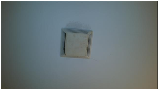
9.4 Item 1(Picture) Bathroom Vent
